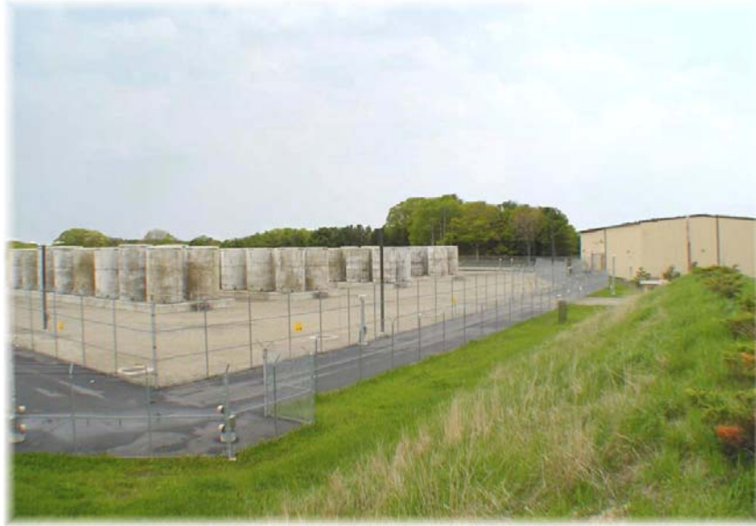
Figure 9. Dry cask storage of spent fuel. Two casks typically contain the equivalent of a year's spent fuel discharges from a 1000 MWe nuclear power plant. Comparison of the simplicity of interim spent fuel storage with the complexity of the huge reprocessing complex shown in Figure 6 makes it easier to understand the relatively low cost of interim storage. 87
