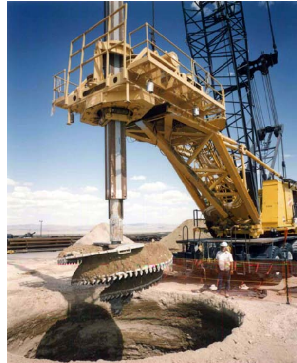
Close-up of drilling equipment for borehole construction
